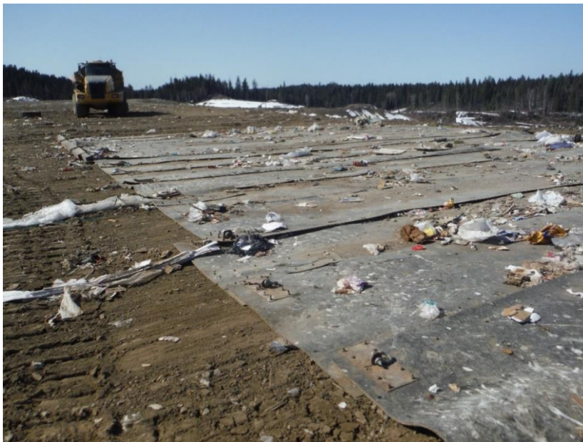
Photo 1 Alternative Daily Cover at the Foothills Blvd Landfill (Prince George)
