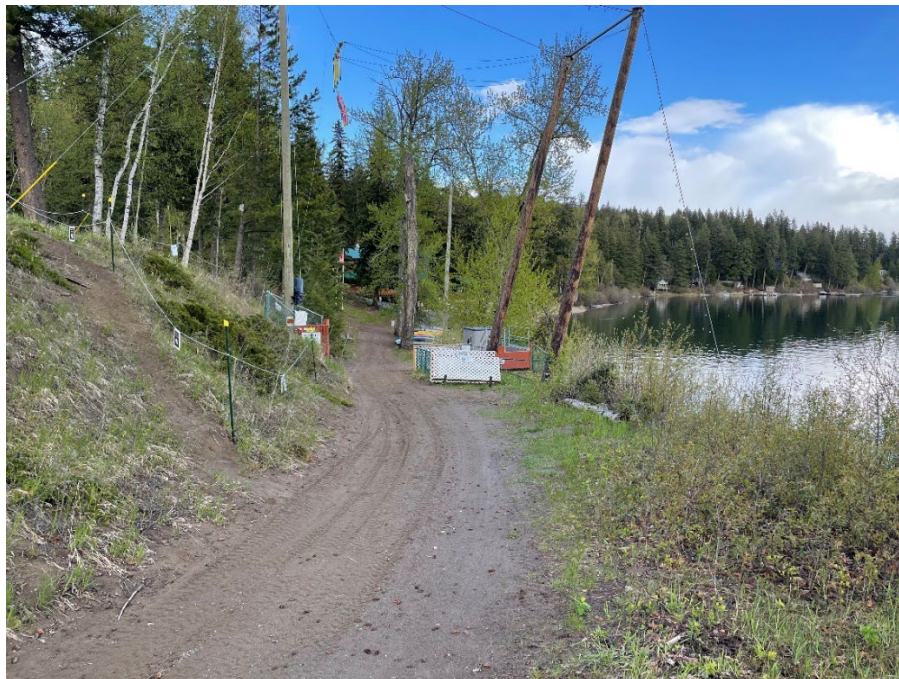
Appendix Photo A-12. East view towards beach. Note common juniper in roped off areas on the left (this is Restoration Site 2) and the shrubs growing on the right within the 15m riparian zone. Three water bars and a sediment trap should be installed on this section of road.
