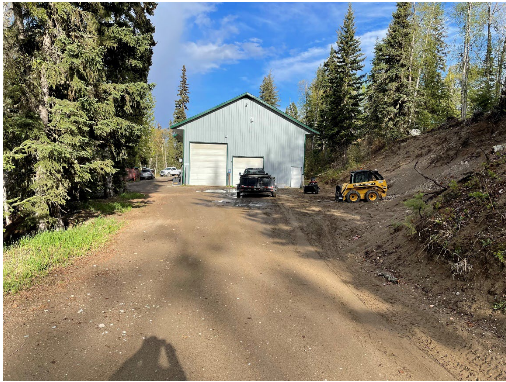
Appendix Photo A-7. Shop and maintenance facility.
