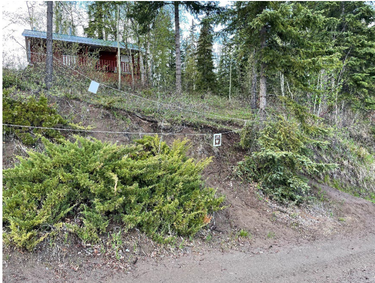
Appendix Photo A-20. Slope on road that leads to beach. This site has been roped off to keep campers out and will be restored with vegetation in the future (Restoration Site 2). Note the erosion and loss of vegetation.
