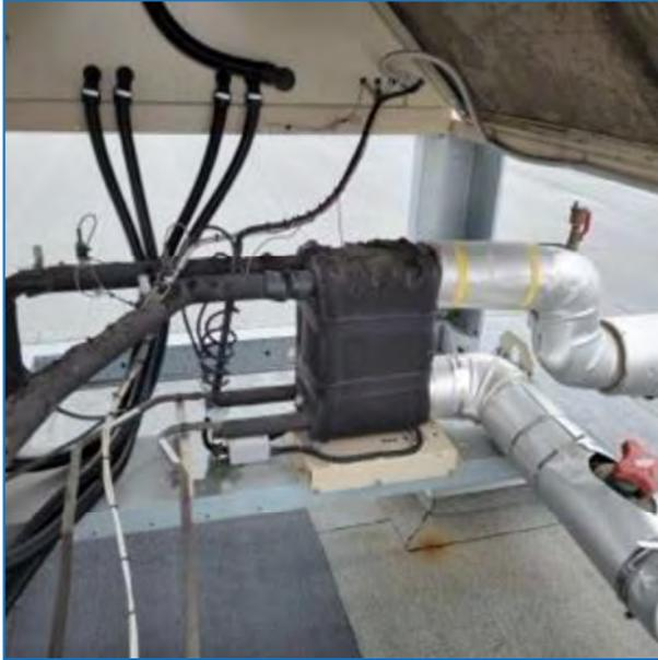
Photo 14 – Chiller Damaged Insulation
