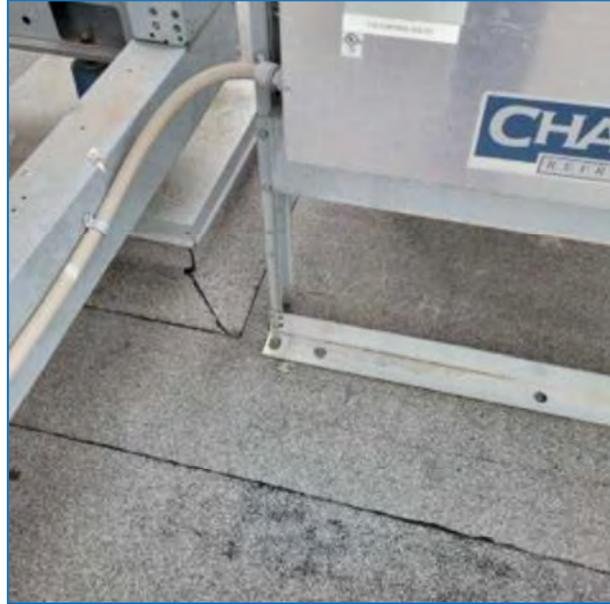
Photo 15 – Fluid Cooler Missing Vibration Isolator
