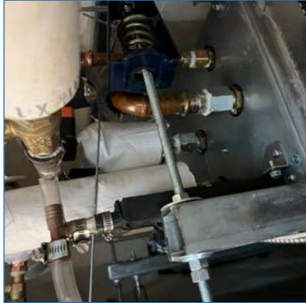
Photo 10 – Piping Connections to the Fan Coil
