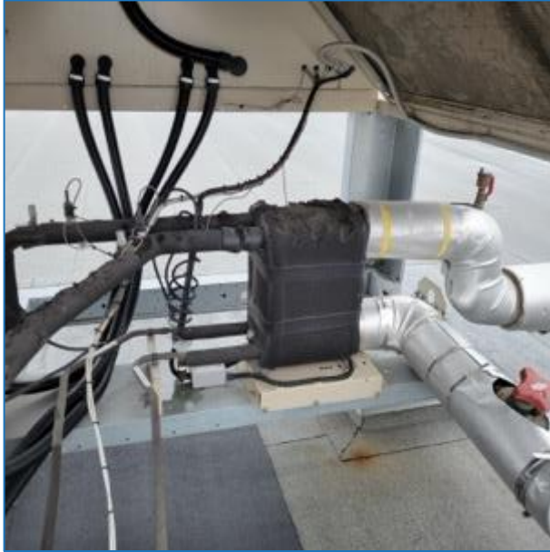
Photo 14 – Chiller Damaged Insulation
