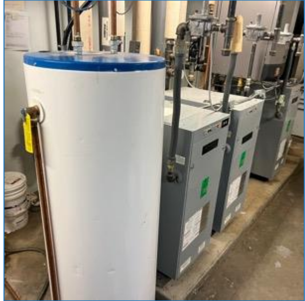
Photo 20 – Domestic Hot Water Heater
