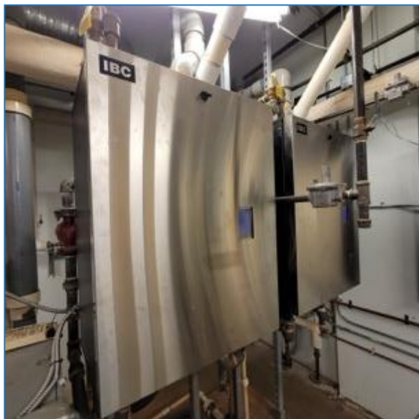
Photo 4 – Hot Water Boilers #1 and 2
