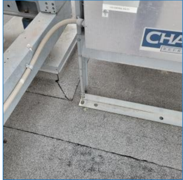
Photo 15 – Fluid Cooler Missing Vibration Isolator
