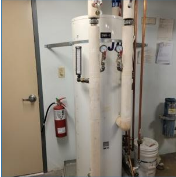
Photo 19 – Domestic Hot Water Tank DWH-1
