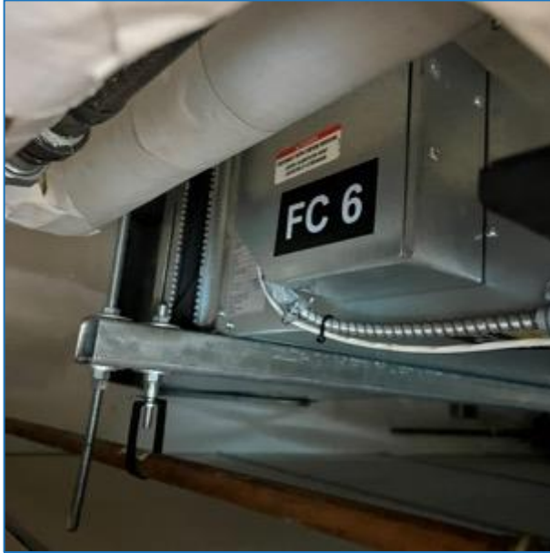
Photo 9 – Typical Fan Coil Unit
