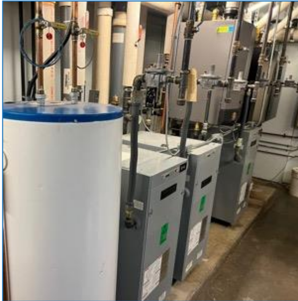
Photo 2 – Hot Water Boilers
