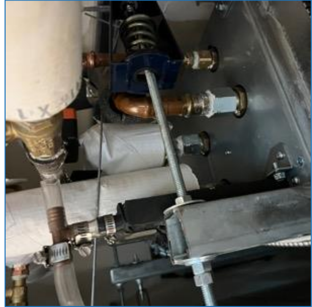
Photo 10 – Piping Connections to the Fan Coil
