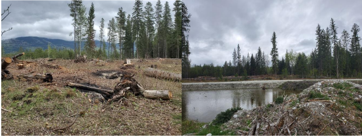
Clearing looking east
