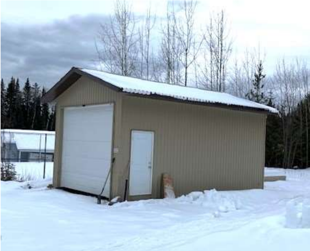
Existing Sno-cat shed
