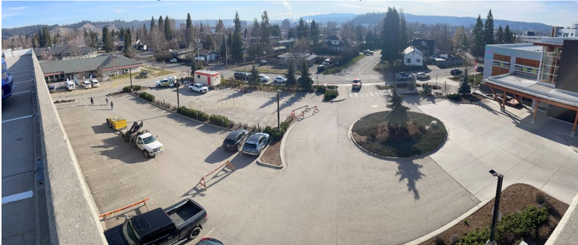
Figure 1: Parkade Construction Site April 2024
