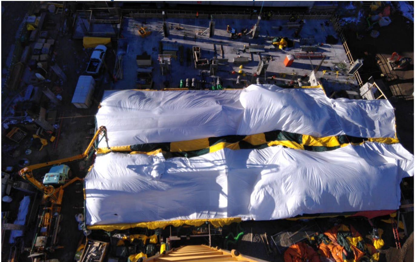
Figure 2: Parkade Construction Site January 2025
